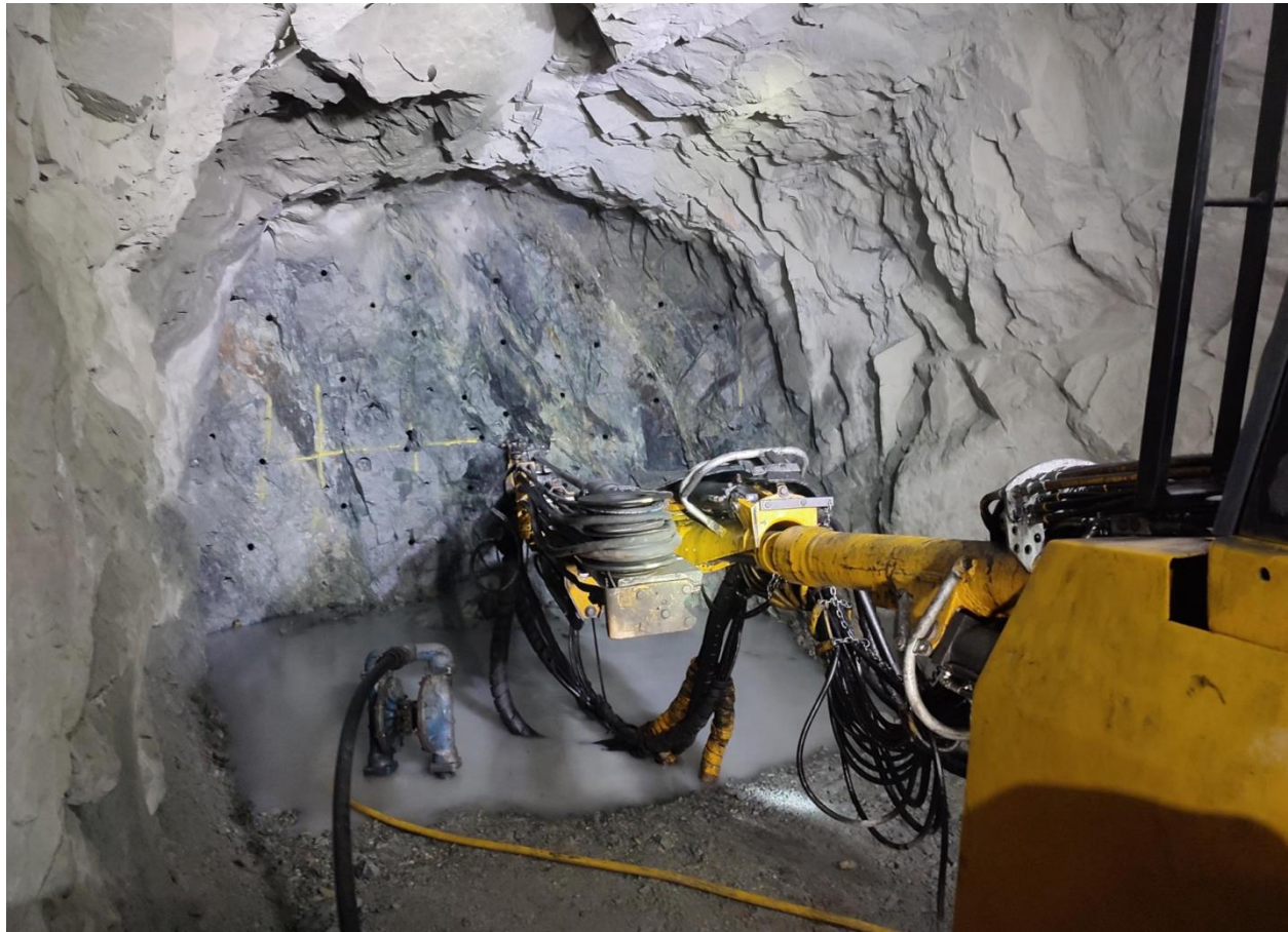
Figure 2. Jumbo Preparing the Advance on the 360 Drift.
