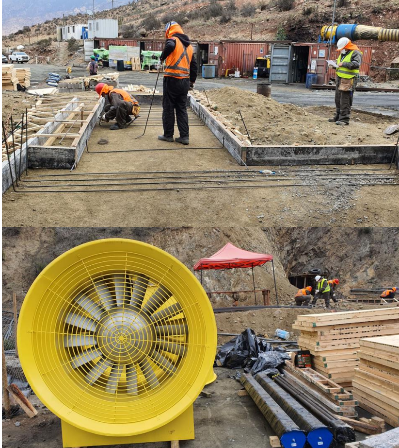
Figure 2. Preparation Work for the Fan Installation
