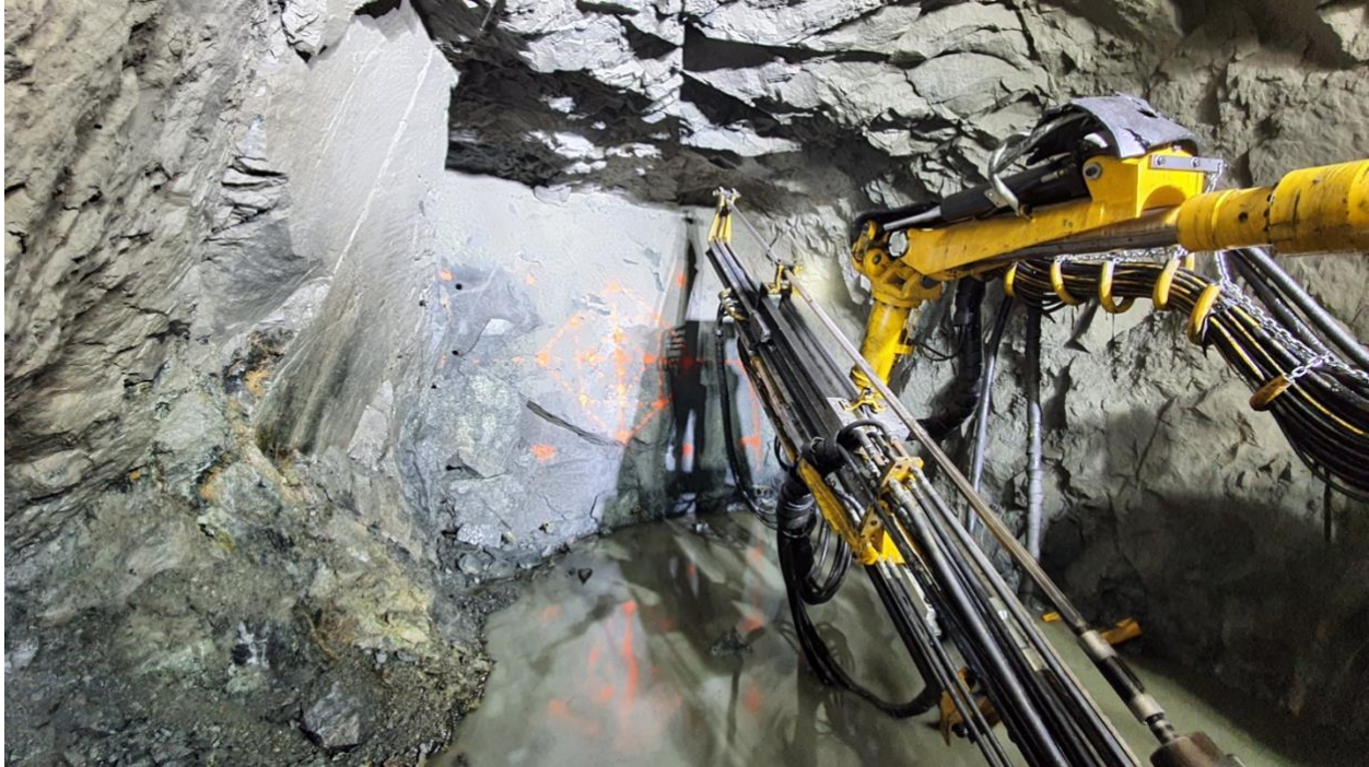
Figure 2. Jumbo Preparing Face for Advancement
