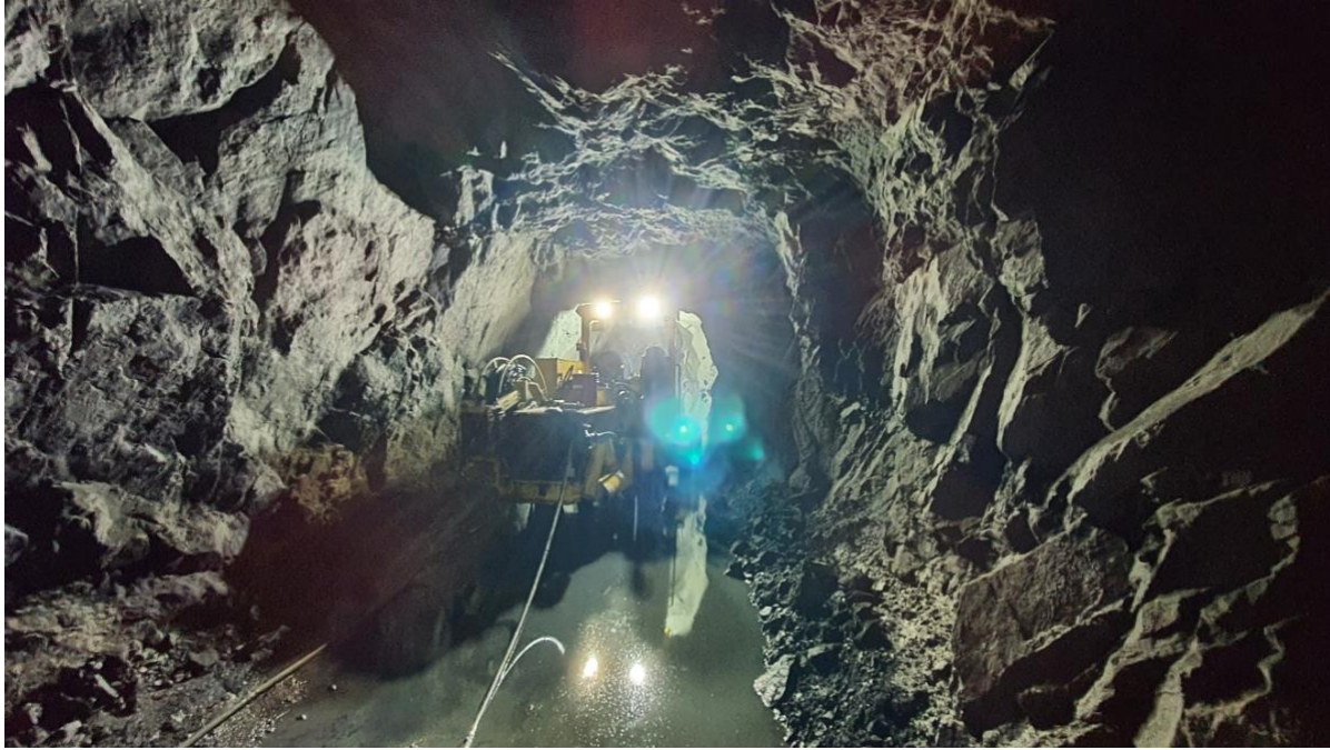
Figure 1. Jumbo Advancing the Hugo Decline to the 376 m level
