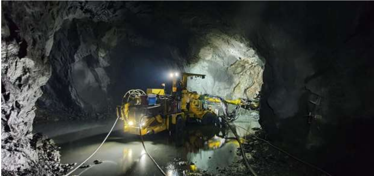
Figure 1: Jumbo accessing 382 m level
