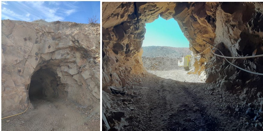
Figure 2: Photos of the Maria Luisa decline entrance
