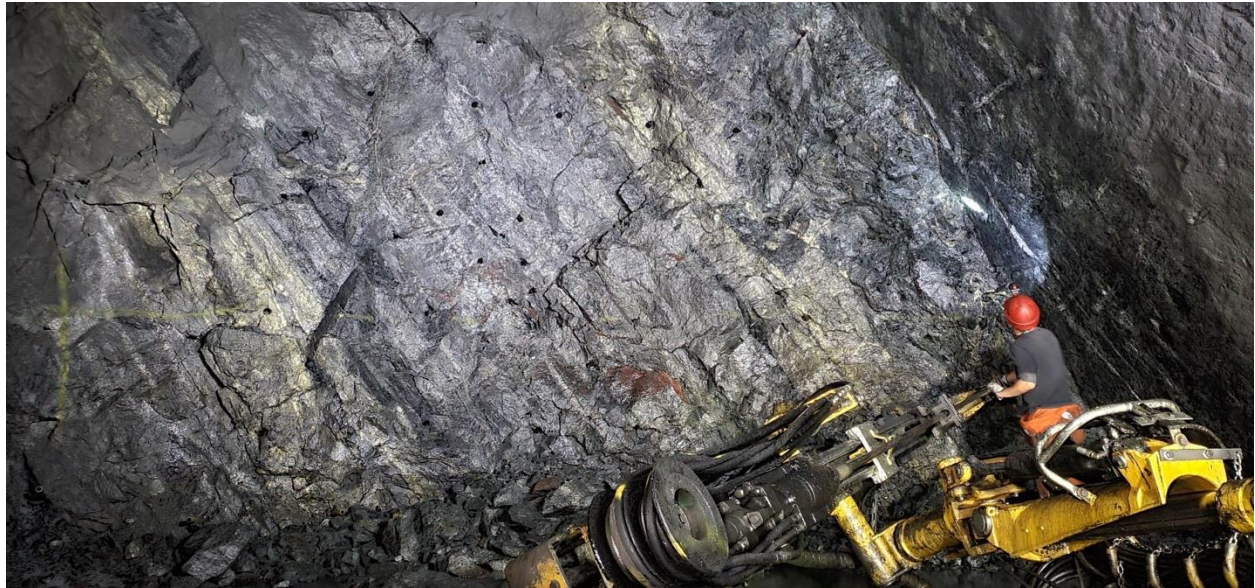
Figure 3. Jumbo in Operation on the 360 m level
