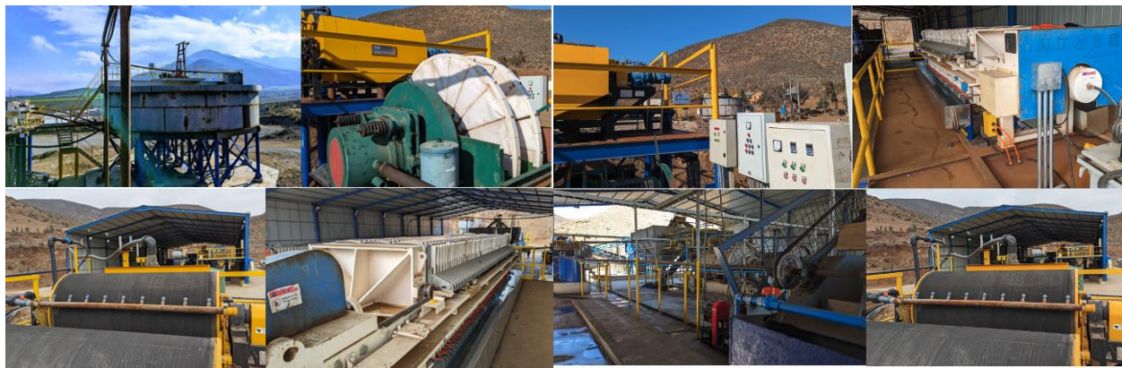
Figure 2. Photos of the El Peñón Facility
